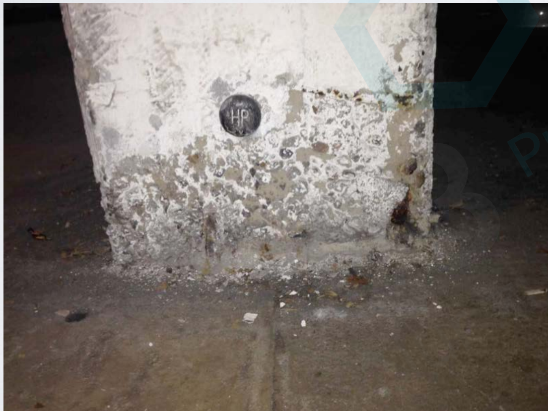
Fig. 25 & 26: Damages in the basement on supports and protection layers
